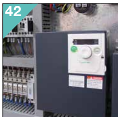
42 Invertor pro plynulou regulaci rychlosti Inverter for variable blade speed.
